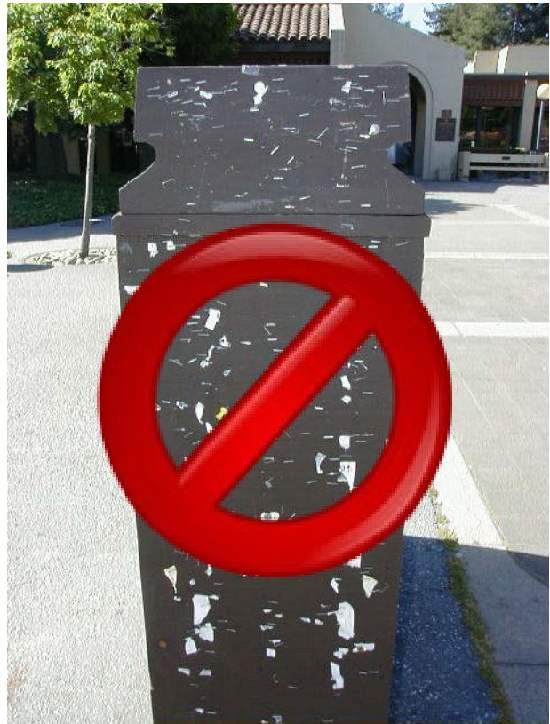
Do not cause damage to college property
